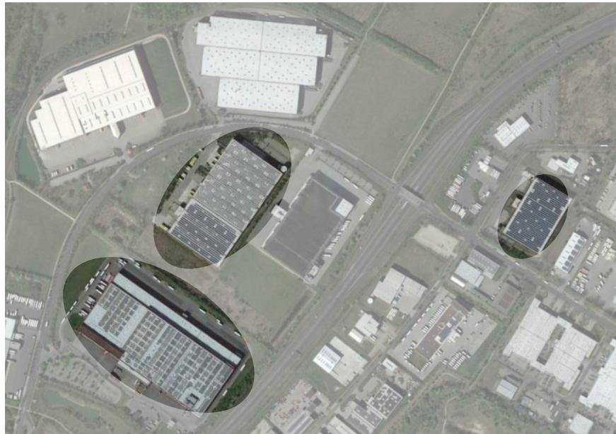
Figure 4-5: Part of logistics hub (Großbeeren, Germany), aerial photo showing roofs of warehouses equipped with PV installations. Source: Google maps
