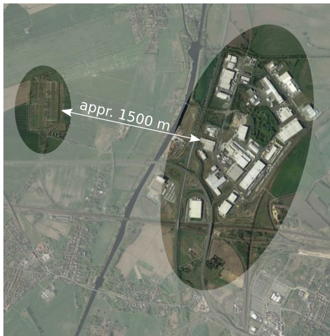
Figure 7. Logistics hub Wustermark, Germany, with a nearby high-voltage transmission substation
